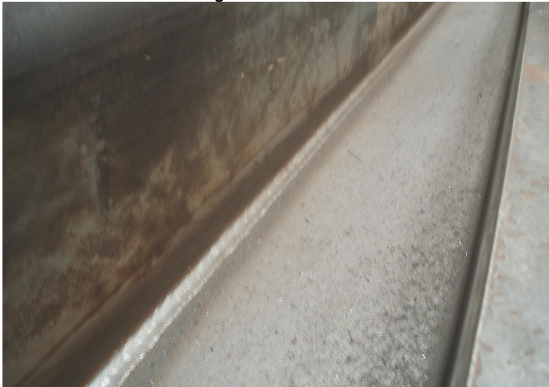
Tony Nuttal – long fillet welds on Osborne's
